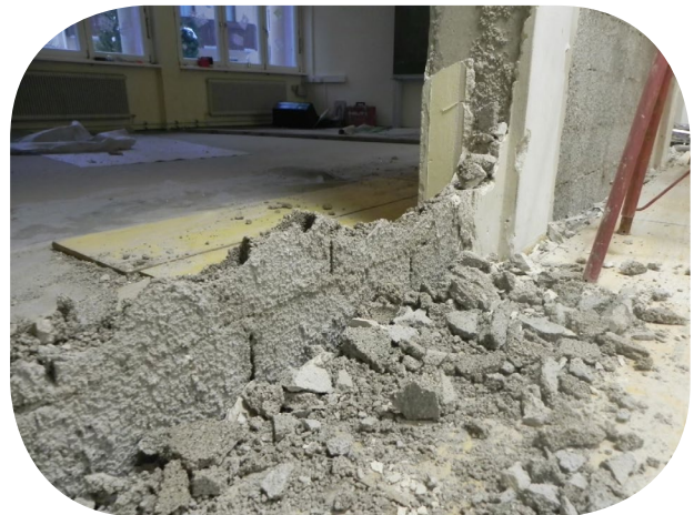
Derrumbando paredes, Zell am See School, Austria
